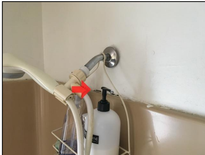
Caulking missing/deteriorated
